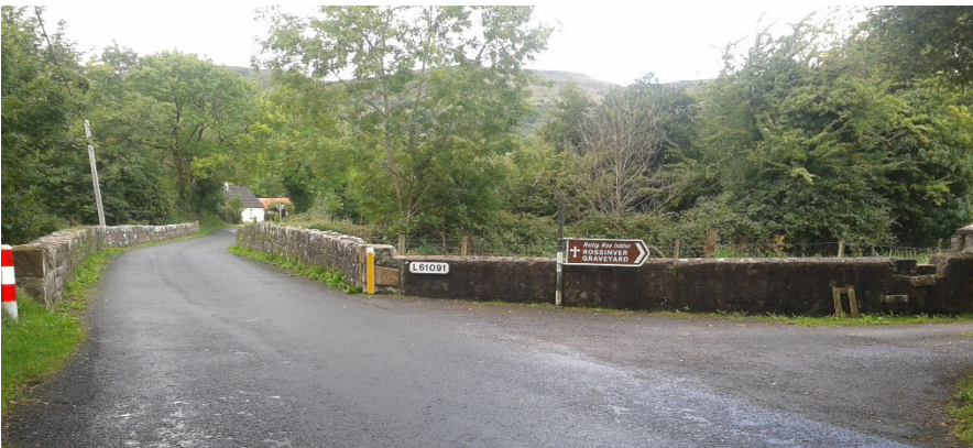
Bridge at Gubalaun near entrance to Rossinver cemetery.
