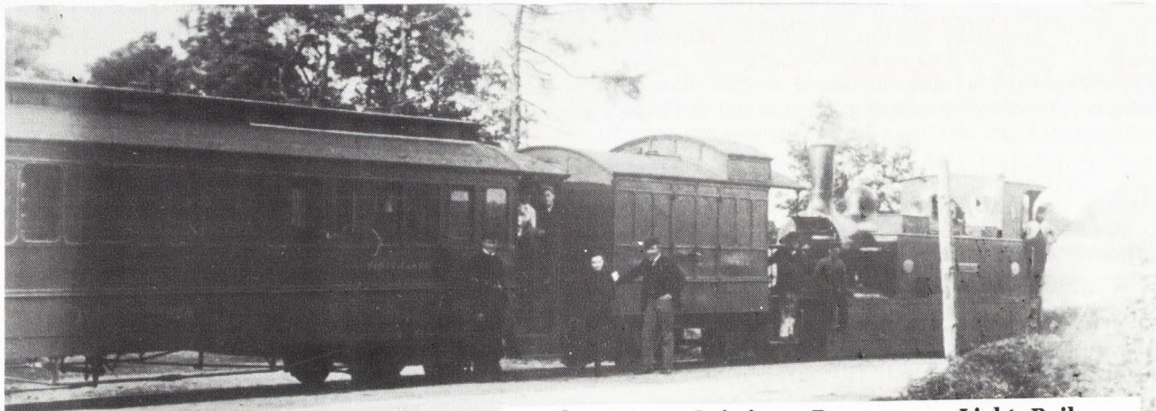
The Cavan, Leitrim Roscommon Light Railway stopped at Annadale (August 1889).
