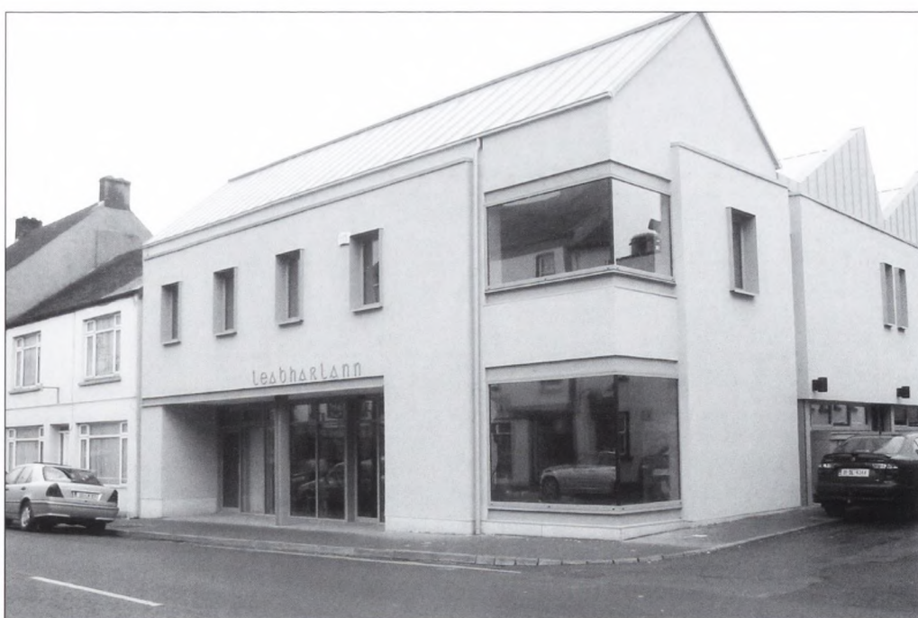
New County Library Headquarters & Ballinamore Branch Library.
